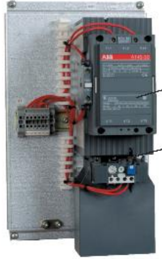
D.O.L starter with contactor and O/L relay
