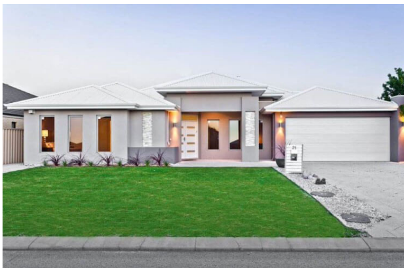
Fig. 5. Painting the roof of the house white.
