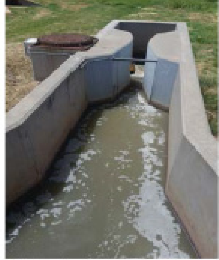
b) The V-notch used to measure the received waste-water
