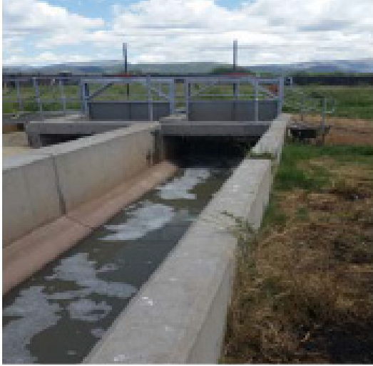
a) Wastewater is received here and physical debris is manually removed
