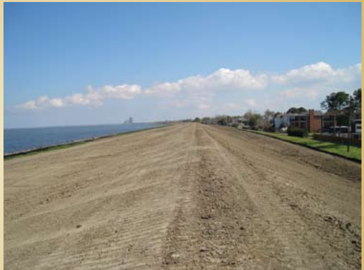
Recent upgrades that raised the height of this earthen levee increased protection against storm surge in the New Orleans area.
