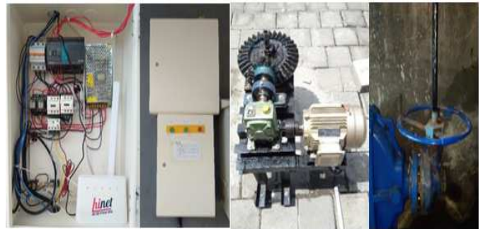
Fig. 4 Realization of the panel and motor gearbox installation on the valve
