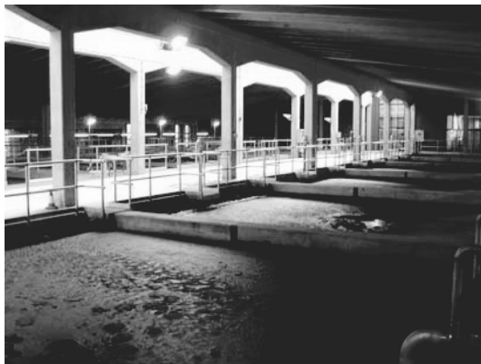
Fig. 5.5 Rectangular flotation tanks.
