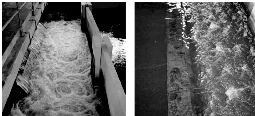
Fig. 3.7 Examples of hydraulic mixers used for (i) rapid mixing and (ii) flocculation at a lowland reservoir treatment works.
