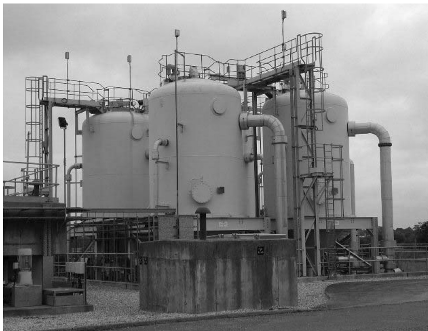
Fig. 8.5 Example of activated carbon pressure adsorbers (image courtesy of Grafham Carbons).
